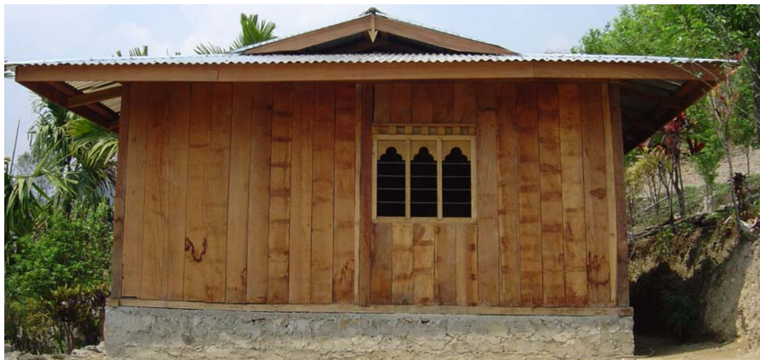
Figure 5: House constructed timber from CF, Sarpang
