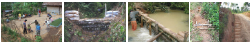
Community action: reduce runoff speed and trap sediment on path road (Photo credits: RUPES Sumberjaya Team)
